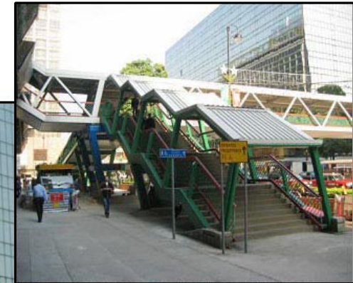
現有行人天橋樓梯 EXISTING FOOTBRIDGE STAIRCASE
