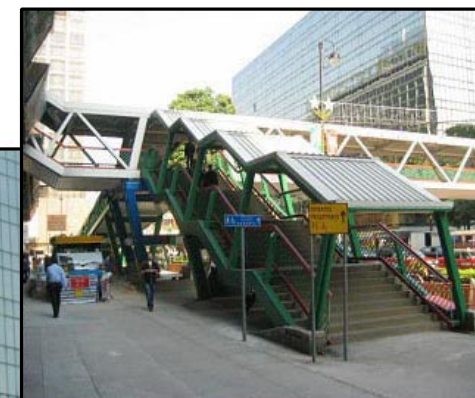
現有行人天橋樓梯 EXISTING FOOTBRIDGE STAIRCASE
