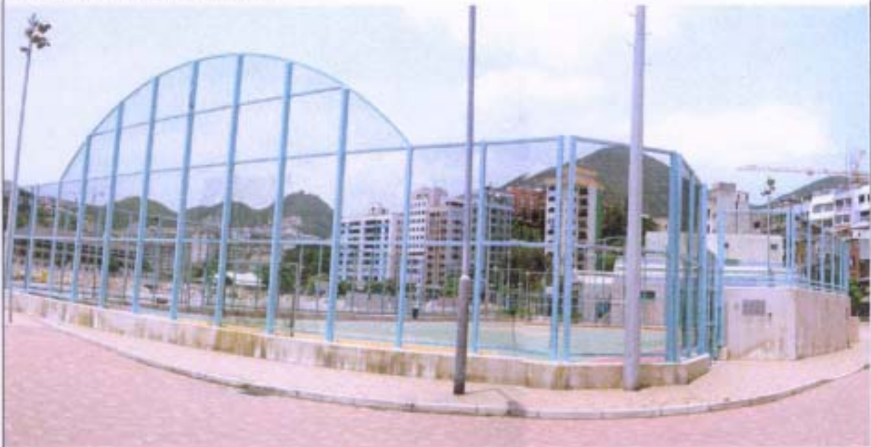
現狀 EXISTING CONDITION
