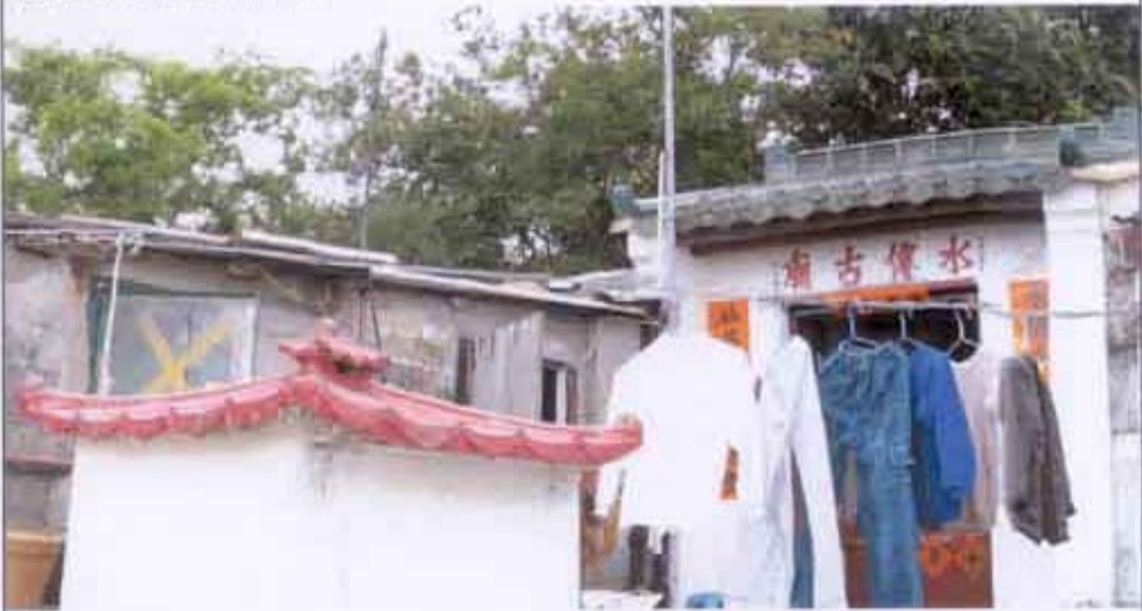
现状 EXISTING CONDITION
