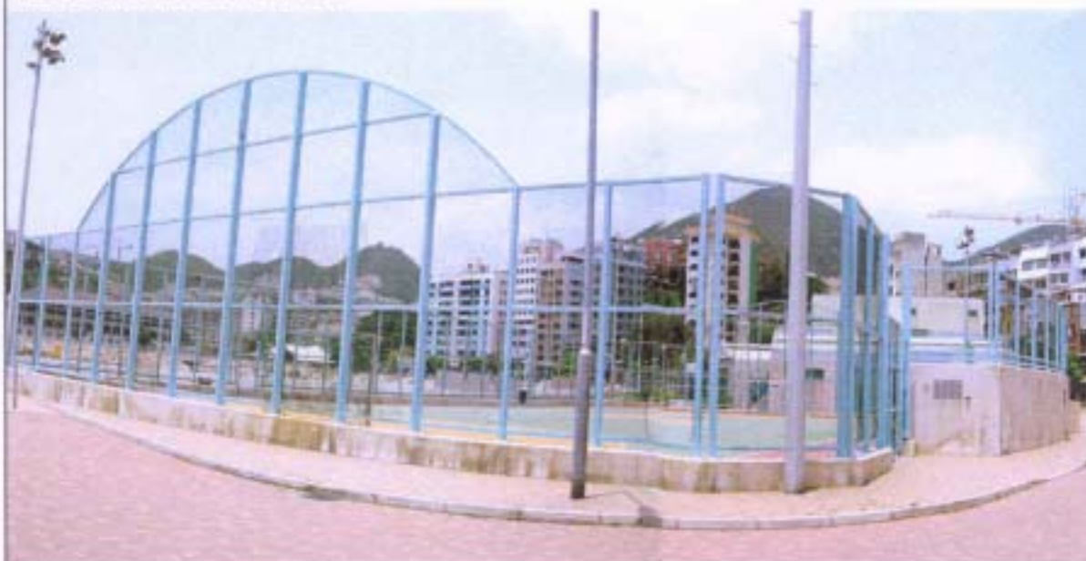
現狀 EXISTING CONDITION
