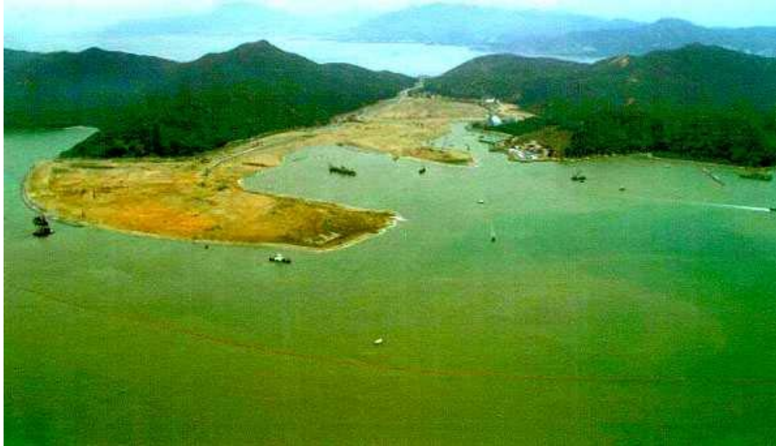
Reclamation Works at Penny's Bay (Outer Bay View)
