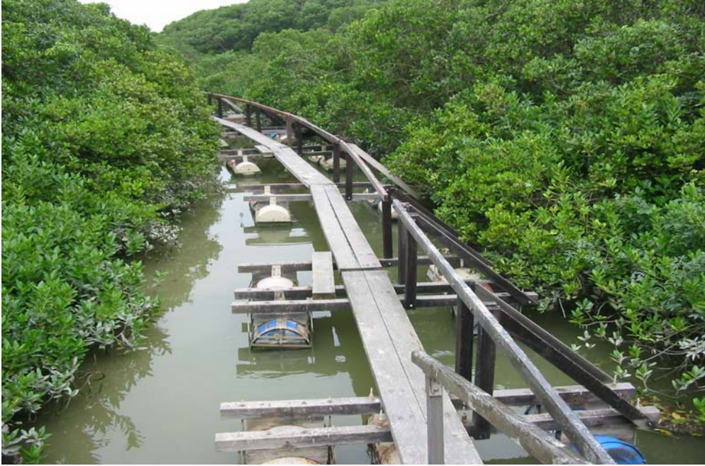
Floating boardwalk at Mai Po provides access to bird hides at Deep Bay
