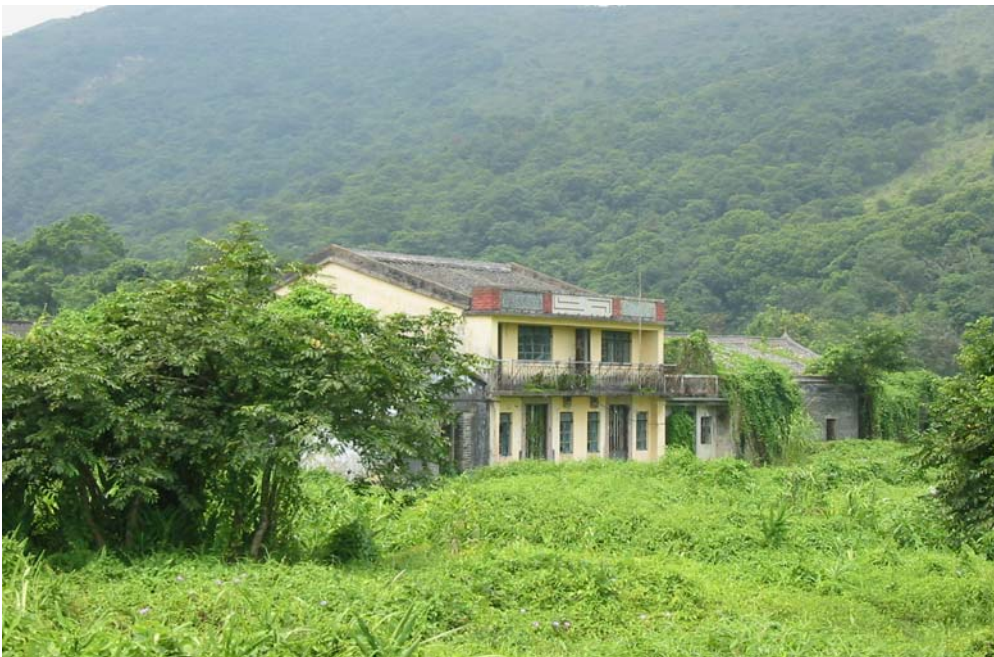
Abandoned but largely intact village house at Sha Lo Tung
